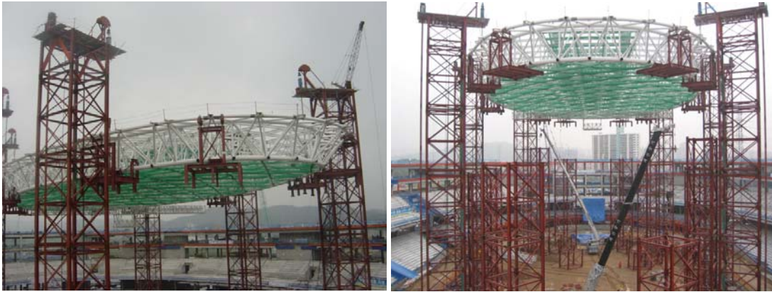
Figure 4. IR lifted up and assembly of ST
