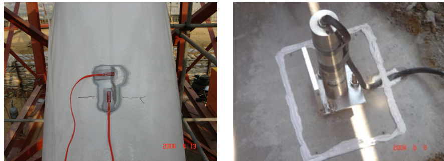
Figure 10. Installation of strain gauges (left) and tilt meter (right)
