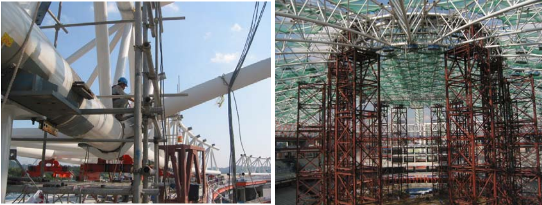
Figure 5. Set up IR on top of ST and installing TR & FTs
